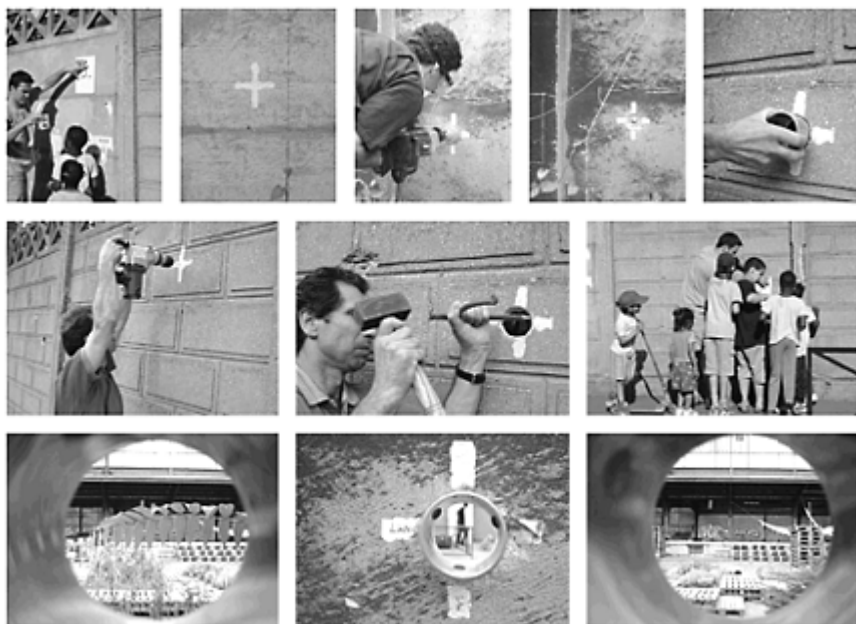
03.07–03.17 – Pipe holes in the enclosure wall, Ecobox, 2003.
